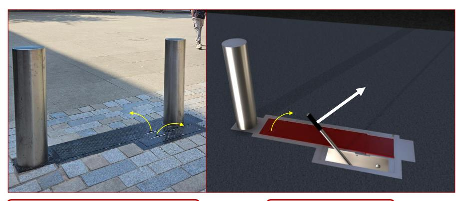
Lift Side Cover and then lift Bollard cover. Unlock hydraulic point and connect lifting hand. Lifting handle is usually retained in bollard cabinet.
