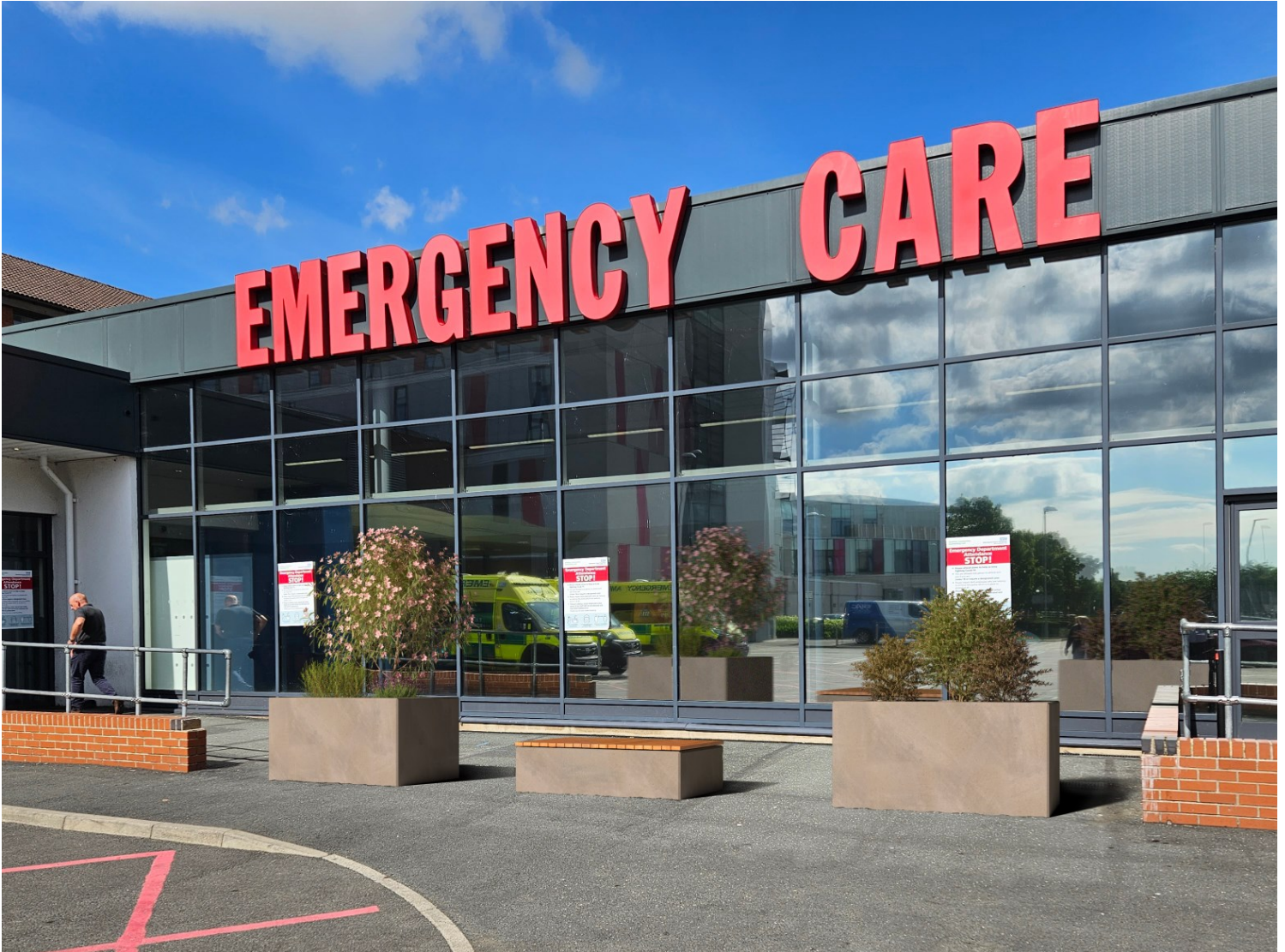
Townscape CT Block Planters with CT Block Deck Seat
